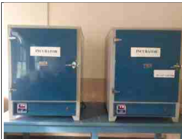
Electrical instruments in New building
