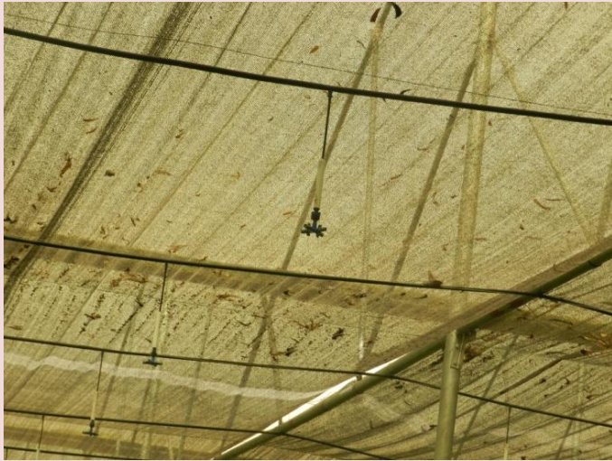
FOG AND MIST GENERATOR FOGGER/MISTER
